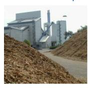
The bio-fuel-powered combined heat and power plant Allöverket, established in 1994, is estimated to have reduced emissions of carbon dioxide in the municipality by more than125 000 tons since 1990. The percentage of bio-fuel is approx. 99 % and it consists mostly of wood chips but also pellets, biogas and bio-oil. The plant is equipped with flue gas condensation.
